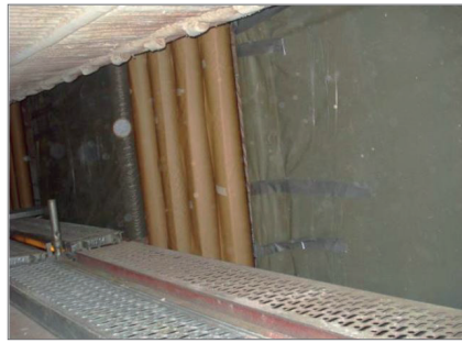
Figure 2 Catalytic tubes covered with paper before application
