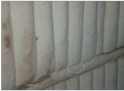
Figure 1 Refractory surface before sandblasting
