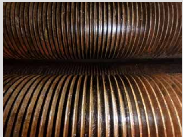
AFTER -Convection Section Robotically Cleaned
